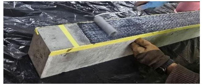
Figure 6. Installation of CFRP by epoxy resin
