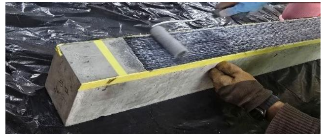
Figure 6. Installation of CFRP by epoxy resin
