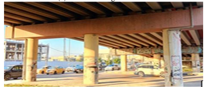
(b) Precast prestressed concrete I-girder
