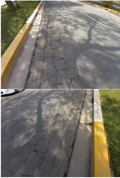
Figure 1. The alligator cracks on the side of the University of Baghdad campus road
