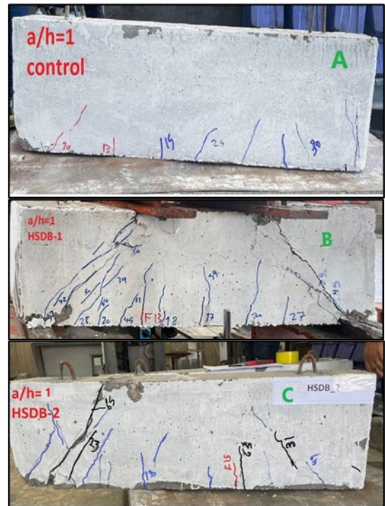
Figure 3. Deep beam specimens at group one ( a/h=1 )
