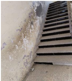
Figure 20. The condition of the finishing materials in the vertical circulation areas of Al-Shaheed Abdul Hakim Al-Safi School
