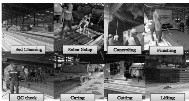
Figure 3. Physical observation of the process flow for precast HCS production
