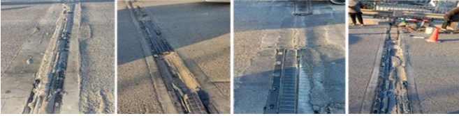
Figure 5. Damages of expansion joints
