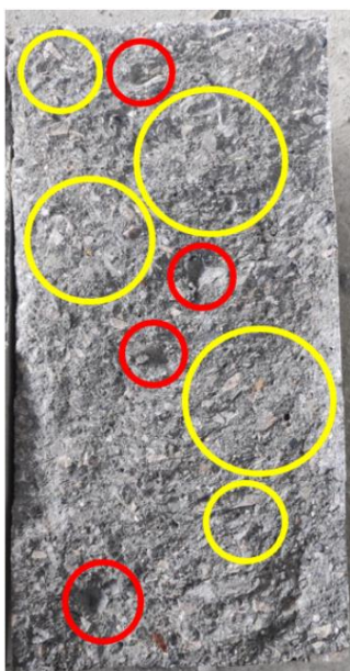
Figure 6. Concrete compression test result: Riven stone (yellow circle) & Detached stone from mortar (red circle)
