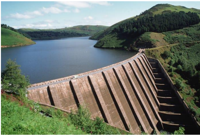
Figure 1. Upper reservoir of storage station
