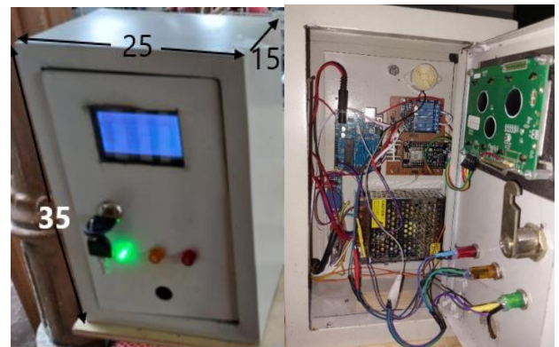
Figure 5. Installation of electronic circuits in the panel box
