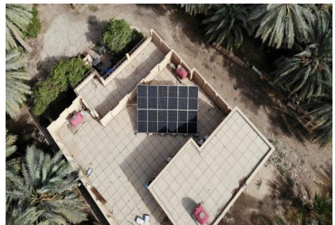
Figure 5. Solar panels prepared for electrical energy generation
