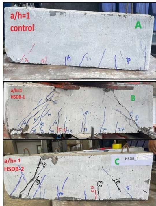
Figure 3. Deep beam specimens at group one (a/h=1)
