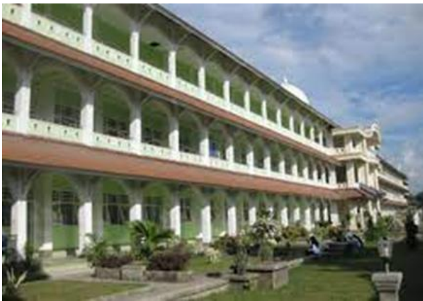
Figure 6. One of buildings at Hamzanwadi University at Pancor, East Lombok Regency
