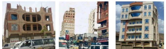
Figure 26. Some buildings in the modern city of Sana'a have lost their identity and character
