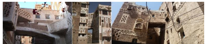
Figure 22. Bridges linking neighbouring residential units in the old city of Sana'a to enhance social interaction and bonding
