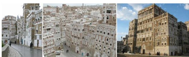
Figure 12. Residential buildings in Old Sanaa Source: [22]
