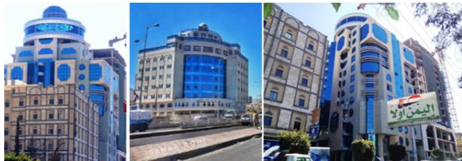
Figure 24. Al-Saidi Tower, modern Sana'a City, with large glass areas
