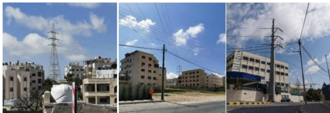
Figure 5. High voltage transmission lines (double circuit lines) passing over urban settlements
