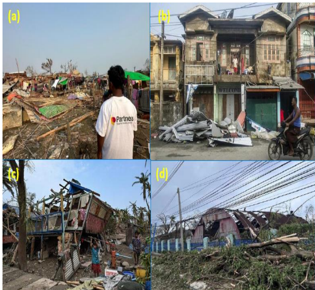
Figure 10. (a) Extensive damage to huts in Rakhine state of Myanmar, (b) Collapsed roof tops, Rakhine (c) damaged houses at Basra camp, Sittwe, Myanmar (Radio Free Asia, and (d) damaged buildings & trees in Rakhine, Myanmar
