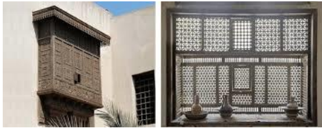
Figure 2. Example of a Mashrabiya in exterior shot (on the left) and in interior shot (on the right) [29]
