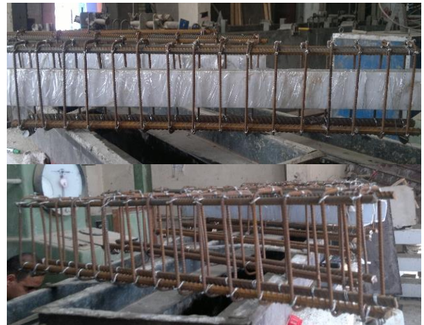
Figure 2. Reinforcing bars and pipe plastic
