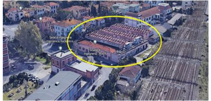
Figure 12. Aerial view of one of the three didactic structure tested (surface: 2134 m 2 , volume: 10296 m 3 and maximum occupancy: 1590 students)
