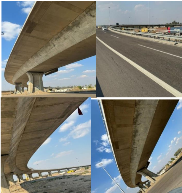
Figure 1. Appearance of horizontal curved box girder bridge
