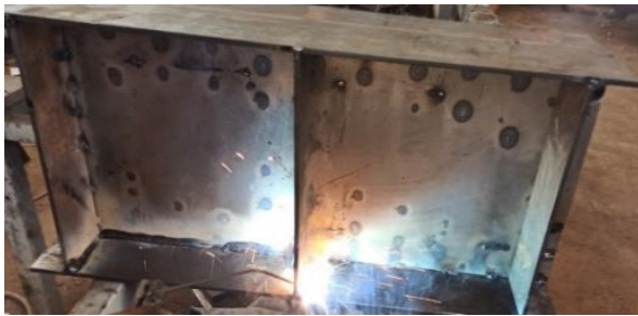
Figure 3. Location of transverse stiffeners
