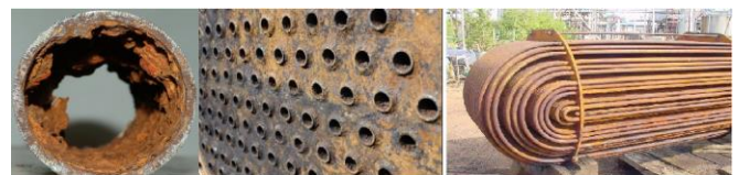
Figure 4. Corrosion in tube and shell of heat exchanger
