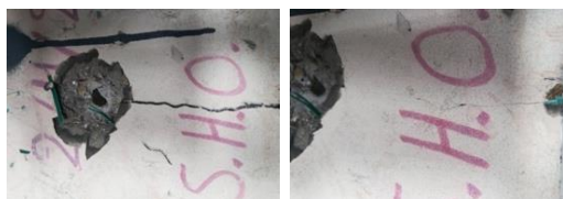
(a) Spalling area and the cracks for the slab that contained 1% NWF of length 50mm
