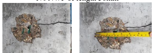
(b) Scabbing area and the cracks for the slab that contained 1% NWF of length 50mm
