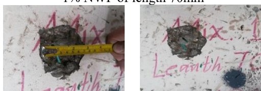
(d) Spalling area and the cracks for the slab that contained 1% NWF of length 70mm
