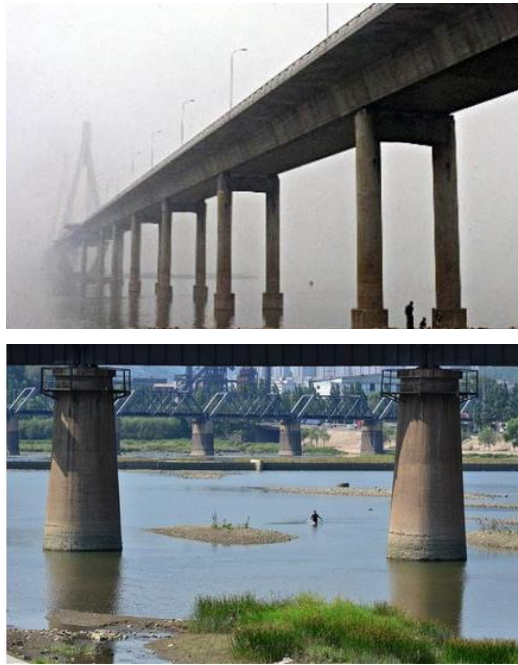
Figure 1. Combined bridge piers
