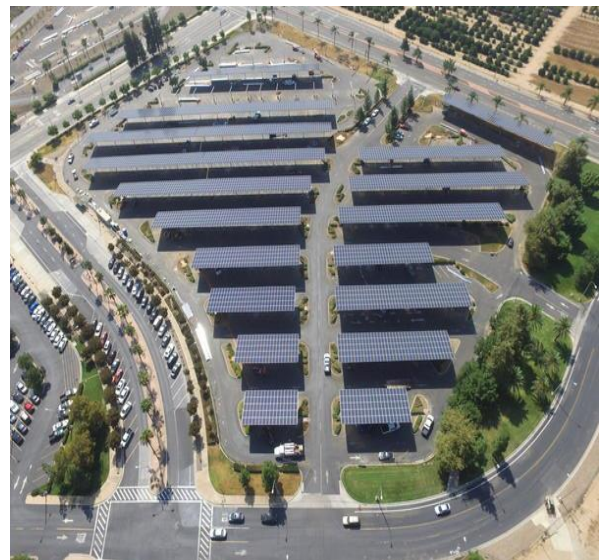
Figure 2. Parking's solar panels (www.ucr.edu/)
