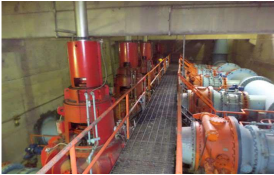
Figure 1. Parallel system of multiple pumping units
