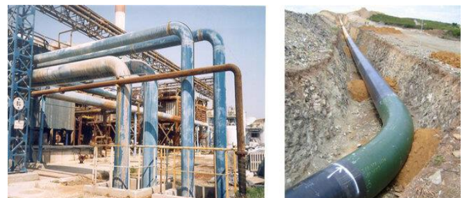
Figure 1. Piping systems in the oil sector demonstrate how elbows erode
