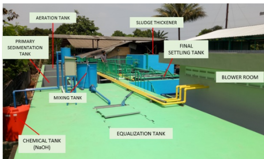
Figure 3. Wastewater treatment facilities for nata de coco
