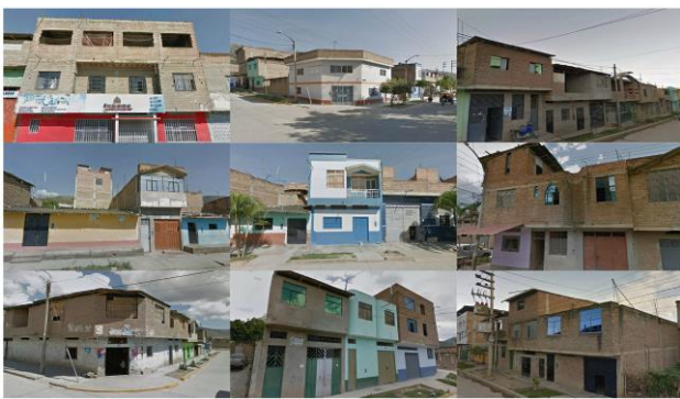
Figure 3. Confined masonry dwellings Jaen, Peru
