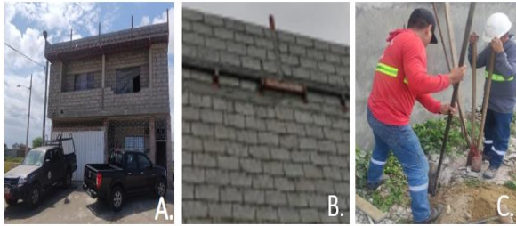
Figure 4. Representative images of the house. A: house in case of study, B: perimeter wall and alignment of the columns, C: manual drilling with hand augers
