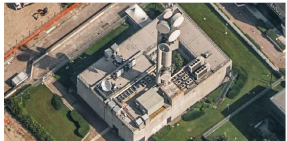
Figure 3. The control building for a main natural gas grid operator
