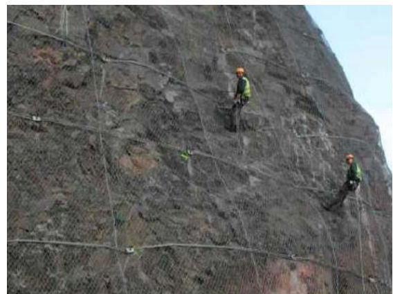
Figure 2. Mesh reinforced with cables
