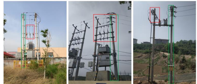
Figure 1. Scale comparison between large equipment and small equipment: the green box is the area of large equipment, and the red box is the area of small equipment
