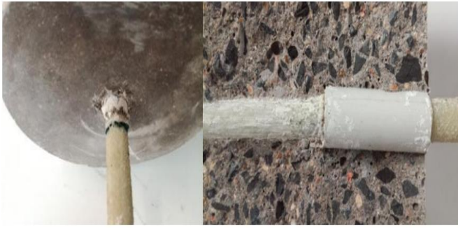
Figure 7. Pull out failure for GFRP rebar 14 ΦS
