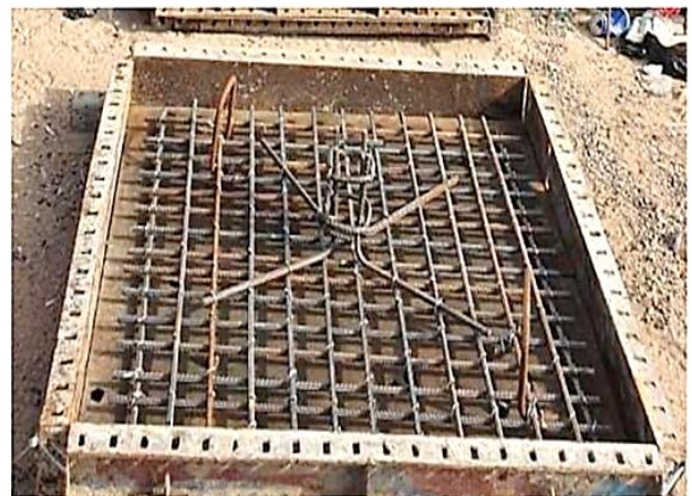
Figure 5. Assembly of reinforcement in formworks
