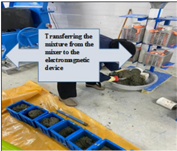
Figure 11. Magnetic concrete processing
