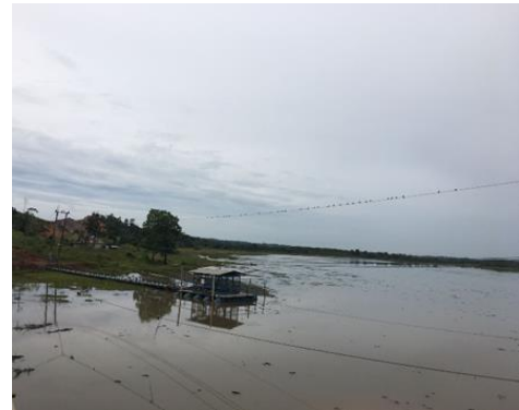
(a) Water suction in the Merdeka reservoir in Samboja sub-district
