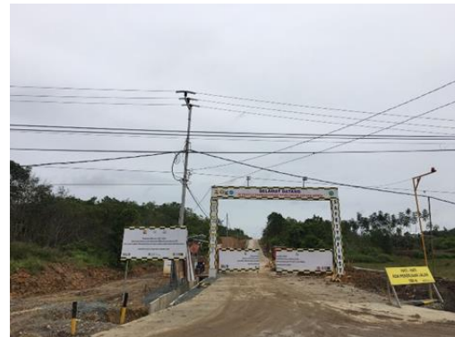
(b) Entrance road for dam construction in Sepaku district
