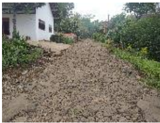
Figure 10. Existing road conditions
