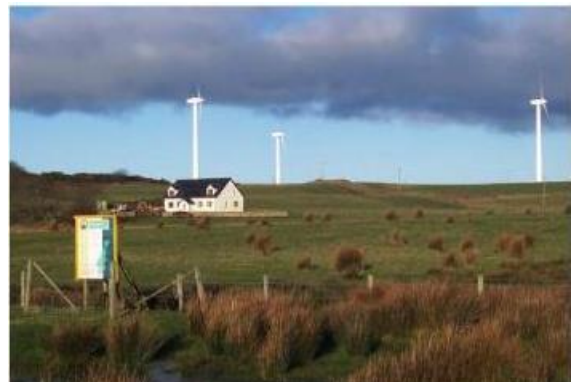
Figure 5. Wind turbine plant
