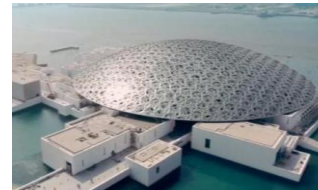
(b) The engineering dome is used as a main source of daylight and at the same time it acts as a giant canopy for the blocks under it ( https://al-ain.com/article/louvre-abu-dhabi-children-museum-opens-june-18 )
