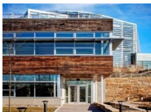
(a) Use solar breakers to prevent glare ( https://cutt.us/KrJqR )
