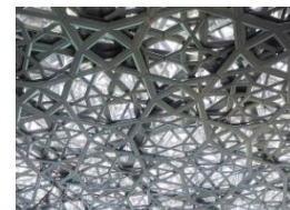
(b) Different sizes of openings designed to determine the quantities of healthy and appropriate lighting ( https://www.pascalls.co.uk/work/leisure-and-hospitality/louvre-abu-dhabi/ )
