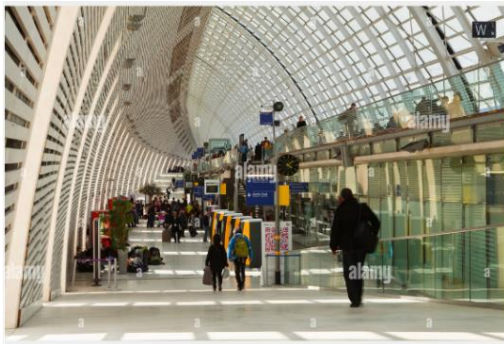
Figure 6. The Avignon TGV station [27]
