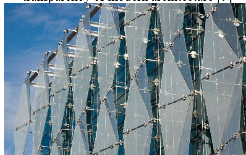
(b) A double-skin glass facade envelops the Knight Center represent duplicated transparency [10]
