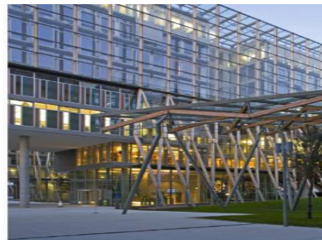
Figure 9. Elm Park development [33]
