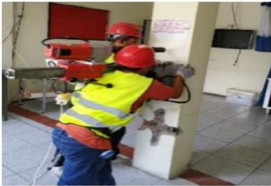
(b) Extraction of concrete cores
