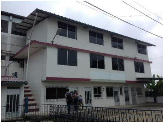
(b) B3 front facade
