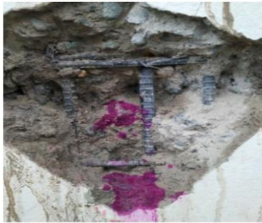
(a) Reinforcing steel
