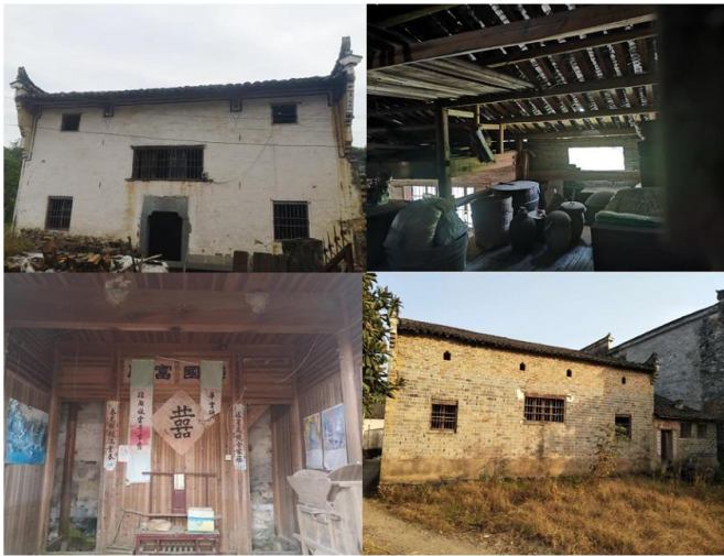
Figure 3. Pre-renovation imagery of the designated project
