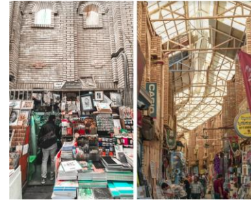
Figure 11. Using brick in facade finishing
