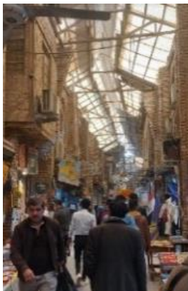
Figure 6. The presence of irregular electrical wires
