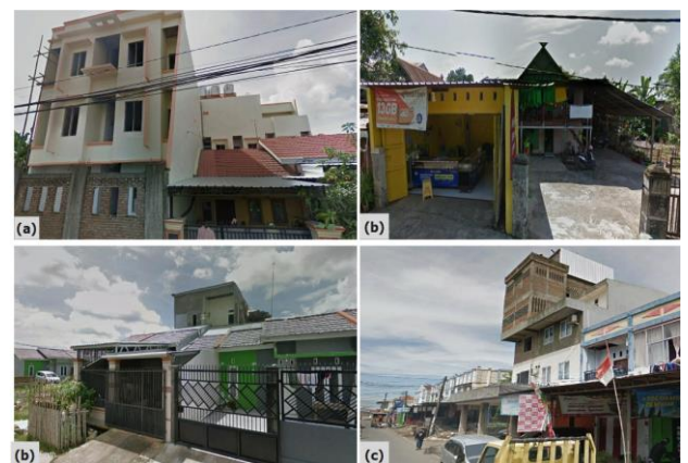
Figure 8. (a) converting and renovating a dwelling to a boarding house; (b) filling the space through the alteration of the yard of a type 21 house and the underbelly of a stilt house, (c) adding floors and roofs to a shophouse complex Source: Author's elaborator
