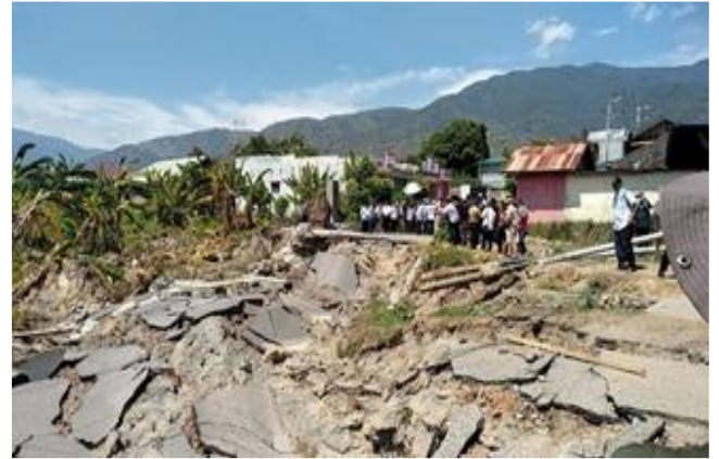
Figure 1. The condition of the liquefaction disaster that occurred in the Petobo area
