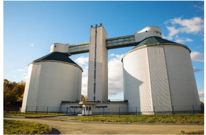
Figure 3. Methane tanks at Northern WWTP
