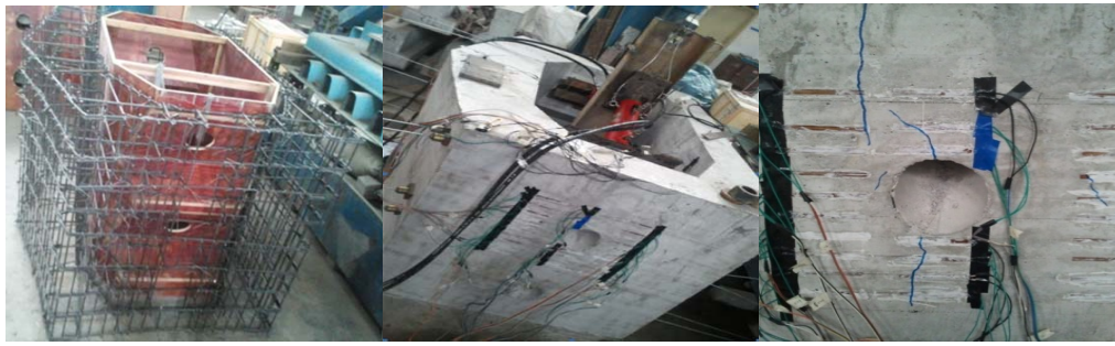
(a) Assembling reinforcement (b) concrete placement (c) crack distribution
