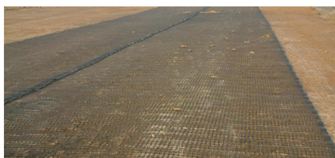
Fig.4. Laying Scene Diagram of Geotechnical Grille
